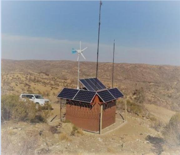
**Figure 2:** Embassy Windhoek's solar-powered repeater
