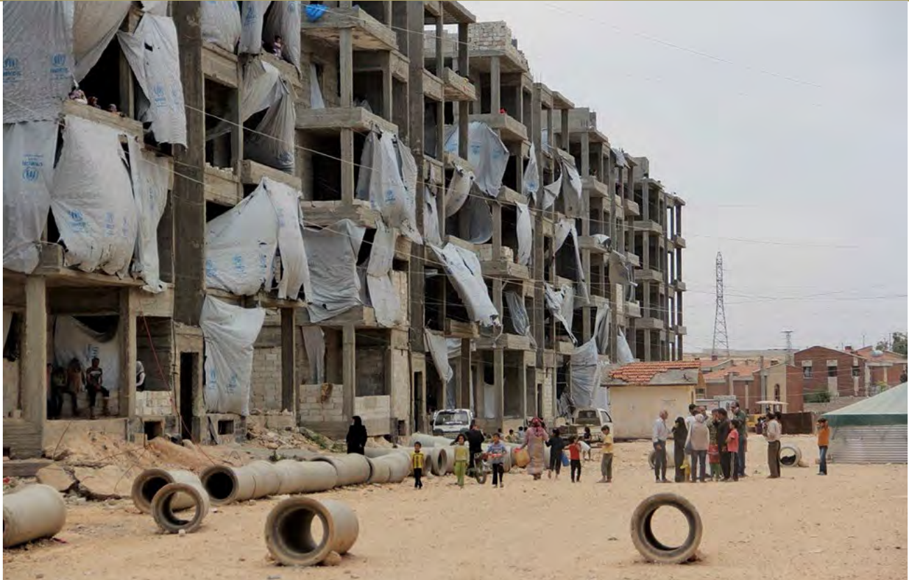
UNICEF and local partners provide water, hygiene, and sanitation services to residents of the Trishin IDP camp in Aleppo city. (UNICEF photo)
